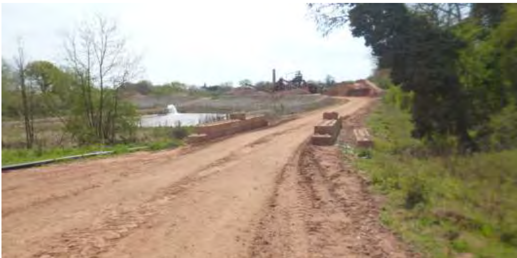
Typical Quarry Haul Road to Plant
